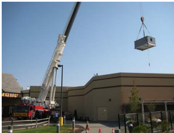
Wildhorse Installs New High Exchange Air Systems
